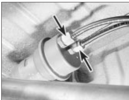
7.5 Fuel pipe connections (arrowed) at the underbody mounted fuel accumulator
